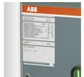
Circuit-breaker characteristics nameplate placed on the front panel.
