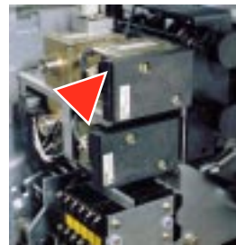
Undervoltage release.
