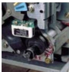
Spring charging geared motor.
