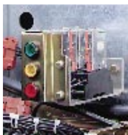
SF6 control device.
