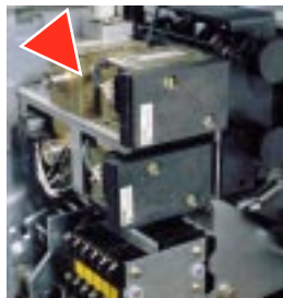
Shunt closing release.
